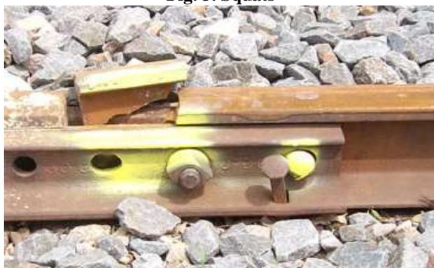
Fig. 4. Broken end rail
