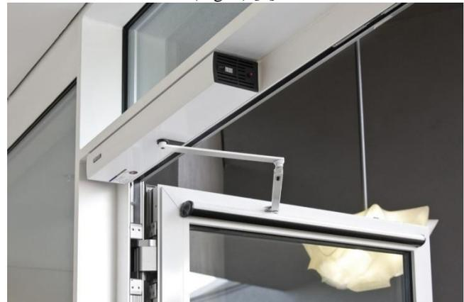
Fig. 2. Automatic drive for opening the access door.
