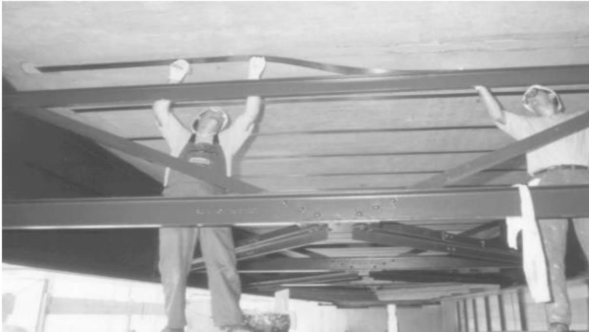
Figure 3.3: (b) Application of prefabricated strips.
