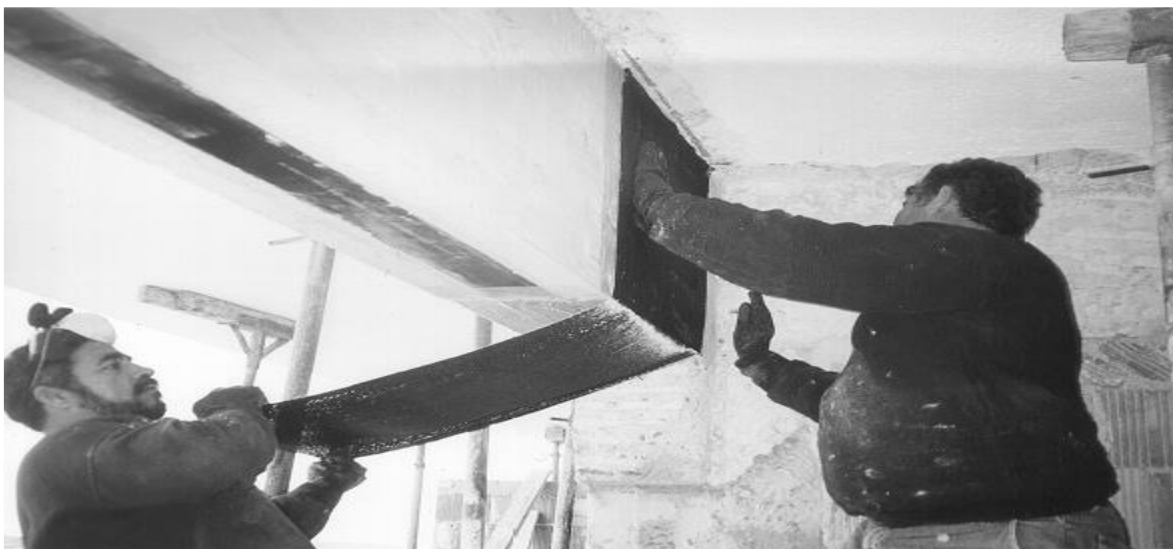
Figure 3.3: (a) Hand lay-up of CFRP sheets or fabrics.
