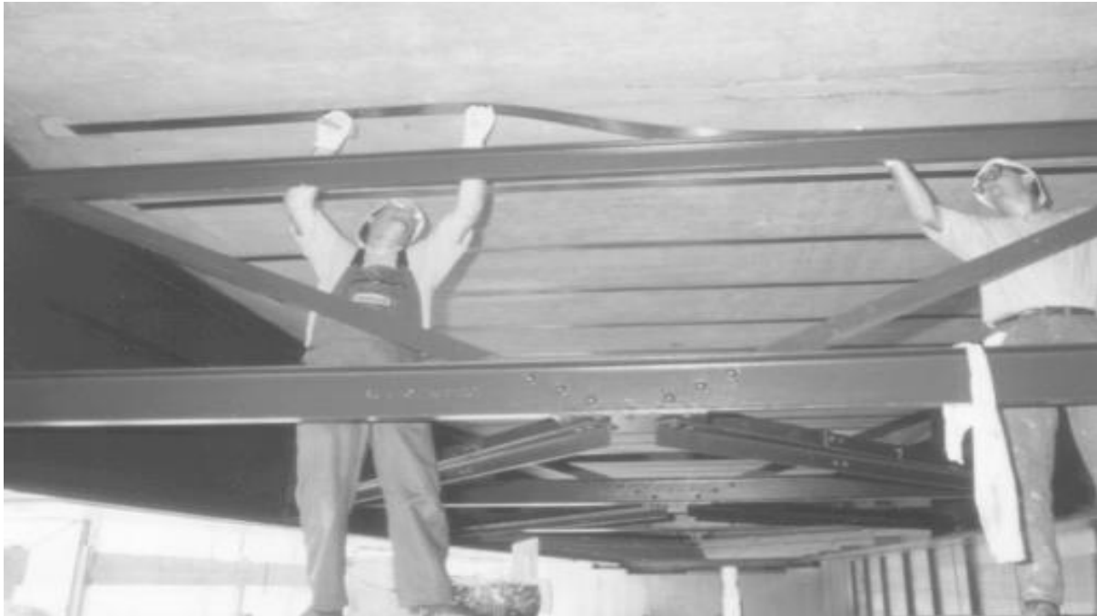
Figure 3.3: (b) Application of prefabricated strips.
