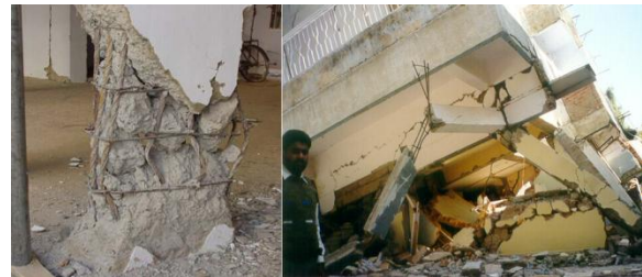
Fig.1 Formation of Column Sway Mechanism
