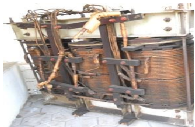
Fig. 1: A view of test specimen.
