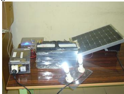
Figure 4d: The whole system during the test (battery, regulator, AC and DC lamps, DC/AC inverter)
