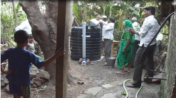
Fig3 : Installation of compact Biogas
