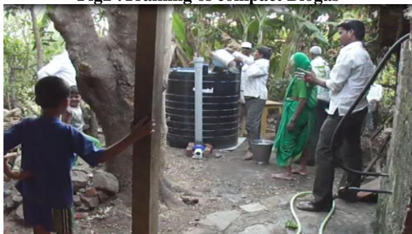
Fig3 :Installation of compact Biogas
