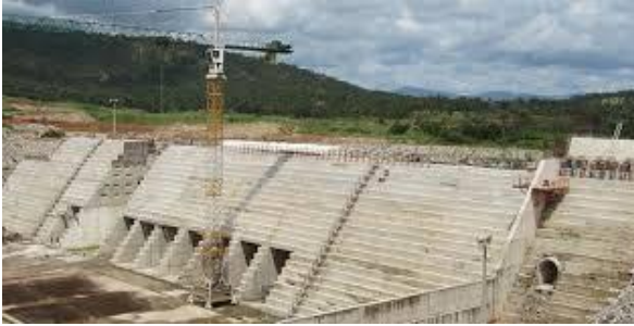
Fig.1: Kashimbilla Multipurpose Buffer Dam in Takum LGA Taraba State, Nigeria
