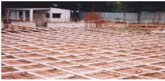
Fig.2 Completed Tendon Layout for the Post- Tensioned Slab system
