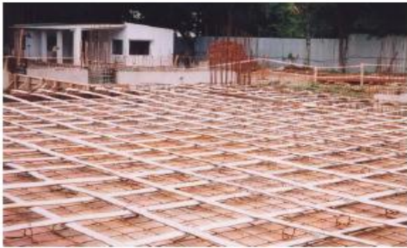
Fig.2 Completed Tendon Layout for the Post- Tensioned Slab system
