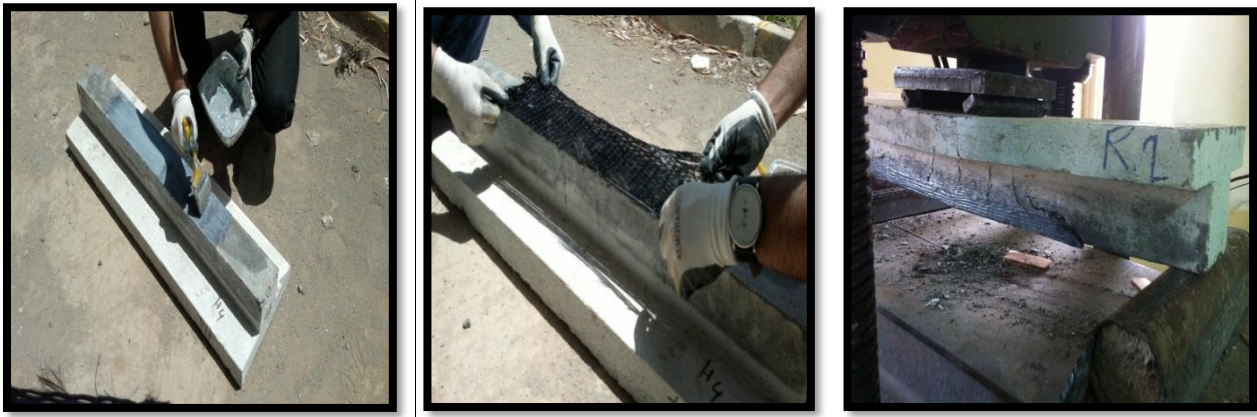
Figure (5) beams rehabilitee.
