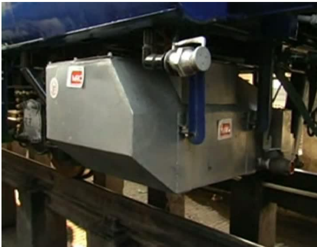
Fig2 : septic tank in Rajdhani express.
