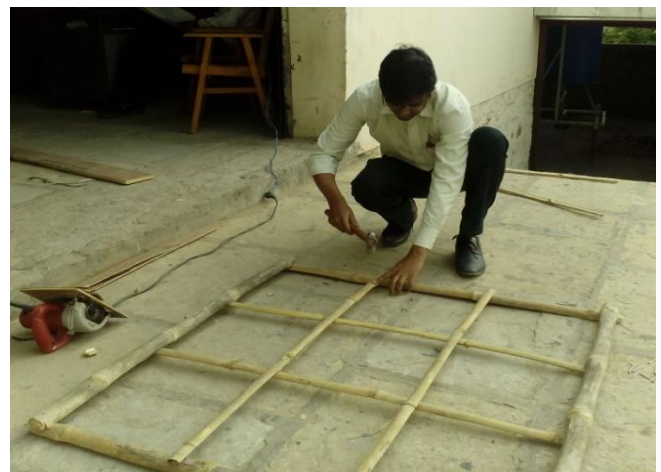
Photo 6: Preparation of Bamboo Panel
