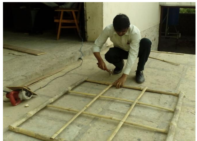
Photo 6: Preparation of Bamboo Panel
