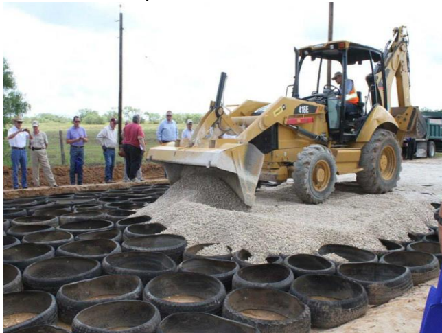
Fig. 2 – Laying of Mechanical Concrete Road (MCR)
