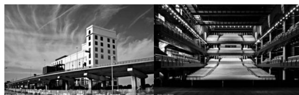
Fig. 18. Abandoned Grain Silo Converted into Arenc Silo Opera House, Marseille
