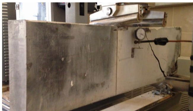
Fig. 5 Failure pattern of ferrocement deep beam BH7.
