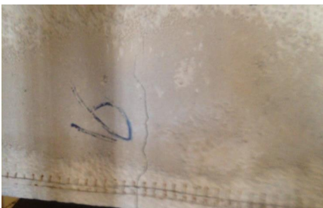
Fig. 7 Failure pattern of ferrocement deep beam BH16.
