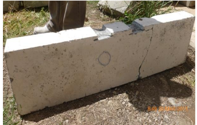
Fig. 4 Failure pattern of ferrocement deep beam B0.
