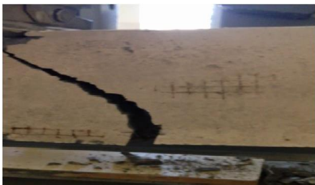
Fig. 6 Failure Pattern of Ferrocement Deep Beam BH12
