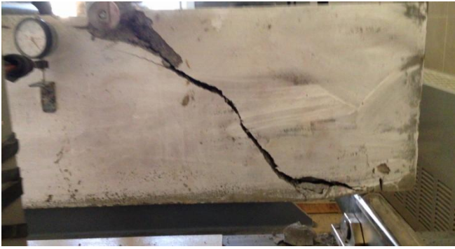
Fig. 8 Failure pattern of ferrocement deep beam BN12
