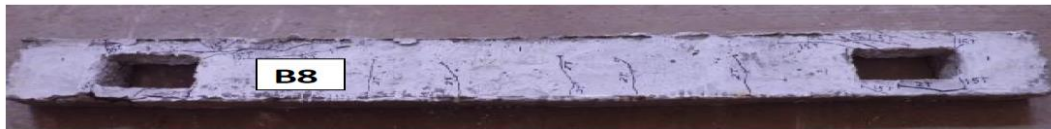
Figure 8.8 Cracking pattern of Beam B8
