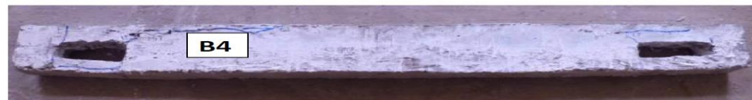
Figure 8.4 Cracking pattern of Beam B4
