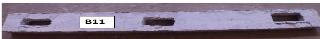
Figure 8.11 Cracking pattern of Beam B11
