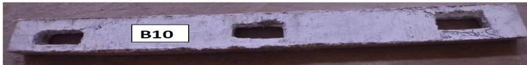
Figure 8.10 Cracking pattern of Beam B10
