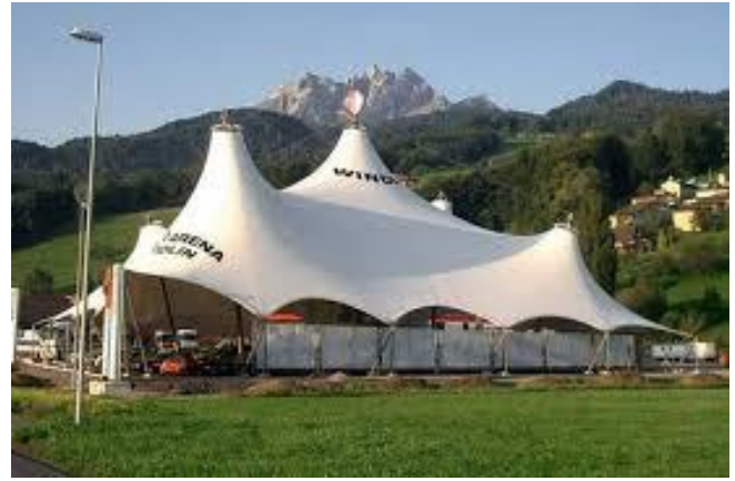
Fig.14. Arrangement of chambers and volumes stretched membrane suspended from the supporting structure.
