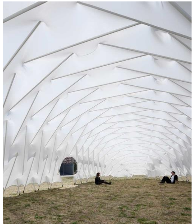
Fig. 15. Space formed under the stretched membrane of tensegrity-structure suitable for placement of chambers and volumes for medical purposes.
