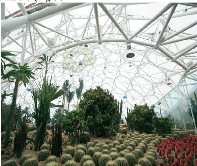
Fig. 5. Passive solar heating. A transparent membrane is stretched over a tensegrity-structure in a greenhouse for exotic plants. Hot water supply for medical purposes with the tubes of the tensegrity- structure.
