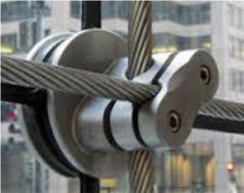
Fig.13. Detail for stabilization of two perpendicular ropes. ( www.thorntontomasetti.com ); (16)
