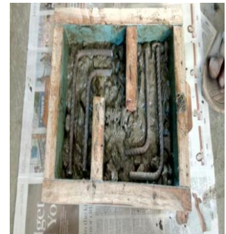
8: Placing of Reinforcement in mould
