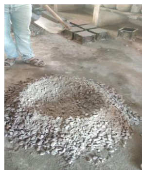
Fig 2: Mixing of concrete ingredients
