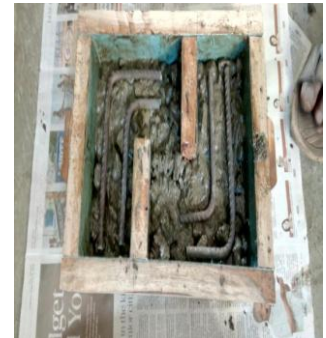
8: Placing of Reinforcement in mould
