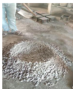
Fig 2: Mixing of concrete ingredients
