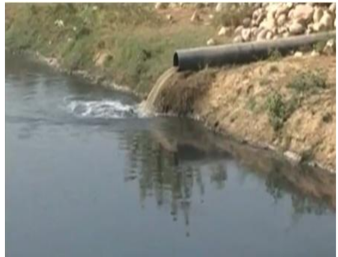
Figure 2 Domestic water is directly released into Satlej near Ropar thermal plant
