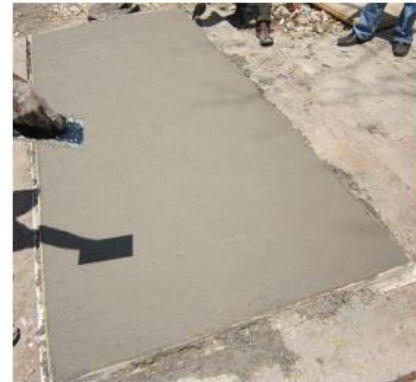
Figure 5: Preparation of mould, Arrangement of filler tiles and Casting of slab
