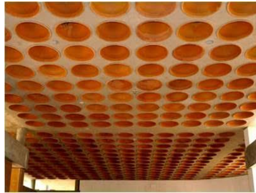
Figure 3: Aesthetic appearance of filler roof slabs
