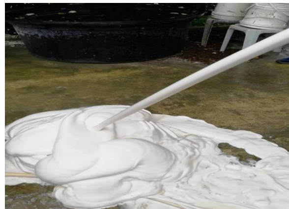
Fig. 3 Production of stable foam through Portafoam TM2 machine
