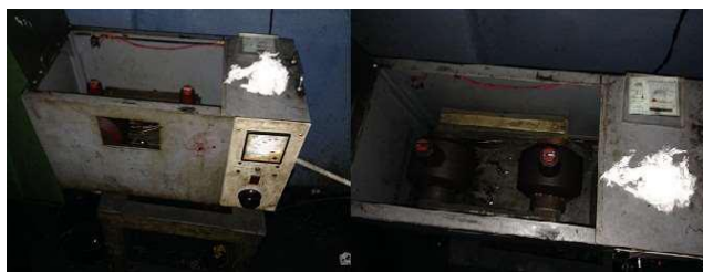
Figure 2: Dielectric Test Equipment at Electrical Sub Station
