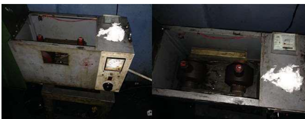
Figure 1 Dielectric Test Equipment at Electrical Sub Station
