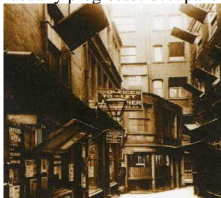
Fig 6. Mirrors remained used to capture day time in narrow streets in London earlier World War II
