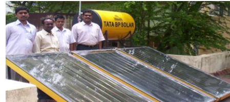
Fig.1.Solar Flat Plate Collector
