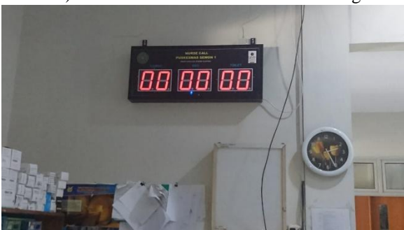
Fig. 1. Installation of a nurse calling device
