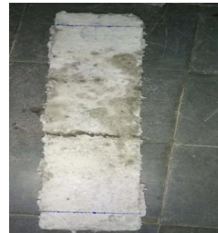
Fig.12. CSRDPFF Beam Specimen after testing
