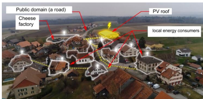
Fig. 7. PV installation and the village (from: Mise au Point, 2018)
