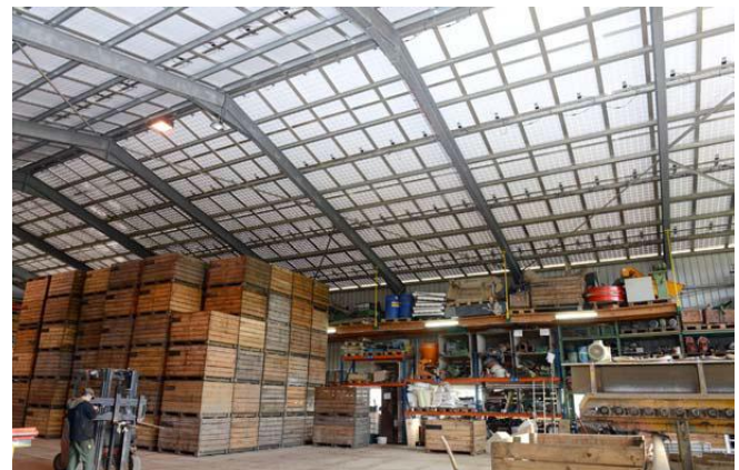
Fig. 6. The transparent photovoltaic panels replaced the cancerogenic Eternit of the farmer warehouse adding brightness to the interior space (from: Mise au Point, 2018)
