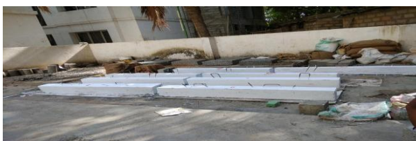
Fig 5: Casted ICSCC Beams
