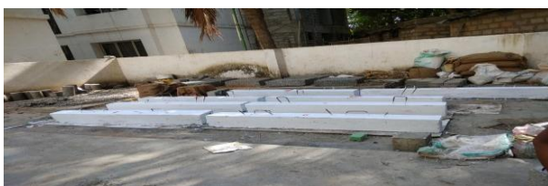
Fig 5: Casted ICSCC Beams
