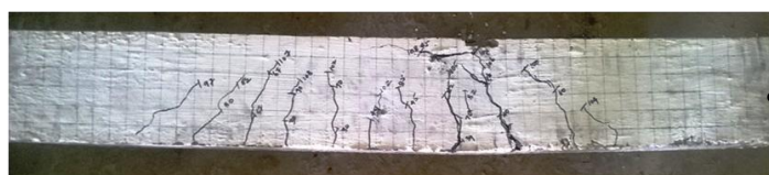
Fig.6 Crack formation in B-2
