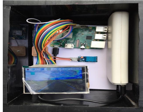
Fig. 7. Hardware components of the non-localized sensor node
