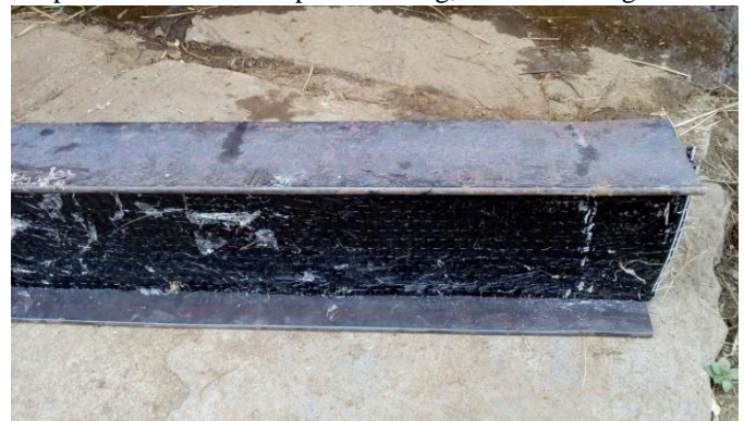
Fig. 3. Web of beam strengthen with CFRP strips
