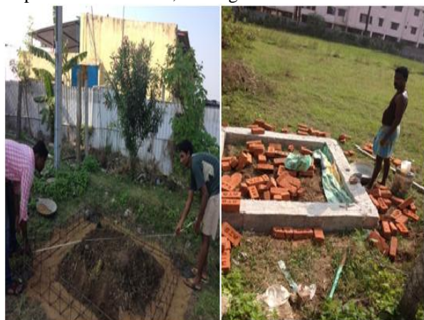
Fig: 2.2. : Placing of reinforcement and construction of plinth beam
