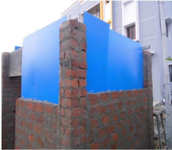
Fig: 2.4 Placing the fluted sheets and Outer-wall construction
