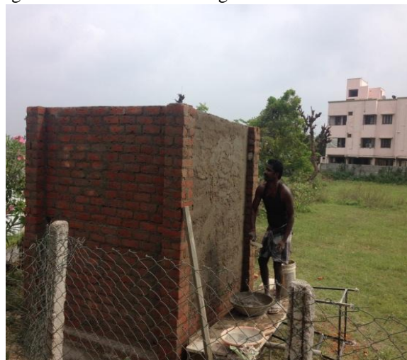
Fig.2.3 Plastering outside of inner wall
