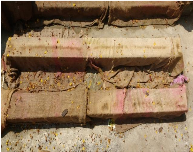
Figure 2: Reinforcement and curing of fiber mixed concrete.
