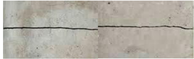
The fig shows the crack made in the Concrete Cube made up of Bacillus Pasteurii
