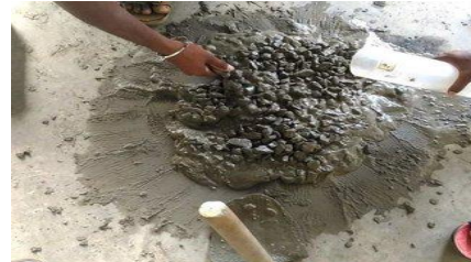
Mixing the concrete
