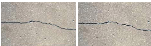
The crack made in the Concrete Cube made up of Bacillus Subtilis
