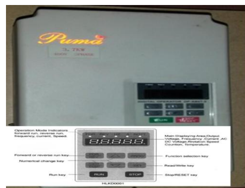
Figure 3 Three Phase Inverter.
