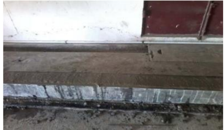
Fig 2 Casting of Beam and surface finishing
