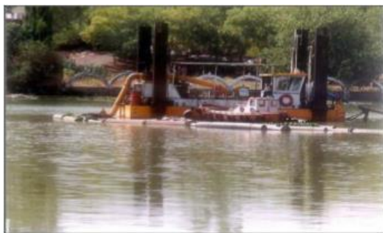
Fig 12 Removal of Silt in Upper Lake Bhopal
