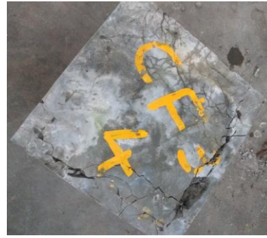
Figure 13 crack observed on four sides supported slab specimen with 0.4% of steel fibre
