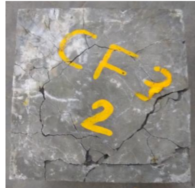
Figure 14 crack observed on three sides supported slab specimen with 0.4% of steel fibre
