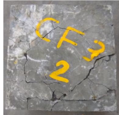
Figure 14 crack observed on three sides supported slab specimen with 0.4% of steel fibre
