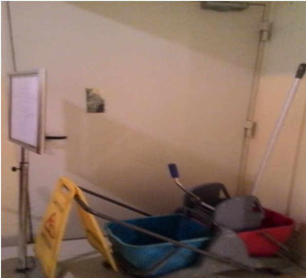
Fig 2. An example of obstructions in the evacuation route.
