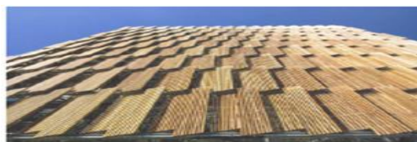
Fig6 : modular porous façade (Forooraghi,M:2015)
