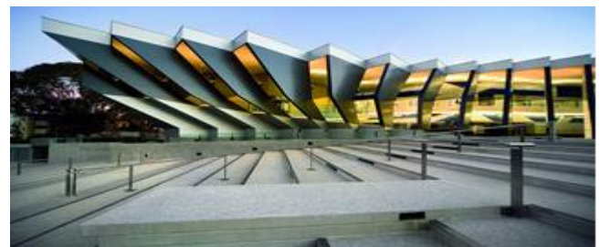
Fig 10:john curtin school of medical research’ by Lyons architecture, the form of façade Controlling the amount of light inside building
