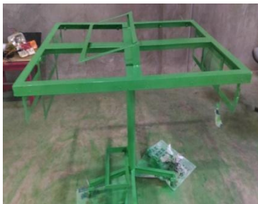
Figure 4. Repainting of frame
