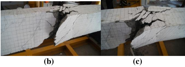
Fig. 10 (a,b,c) Failure of conventional steel reinforced beams due to concrete crushing ( Bp_2m_2F_c )
