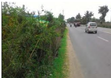
Fig. 12: Inadequate width of shoulder
