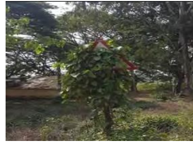
Fig. 14: Sign board covered with vegetation at ch.188.100 Km
