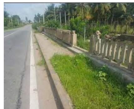
Fig. 18: Damaged parapet
