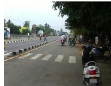
Fig. 16: Poor visibility of Bus stop at ch.197.300 Km
