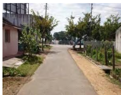
Fig. 11: Lack of sight distance
