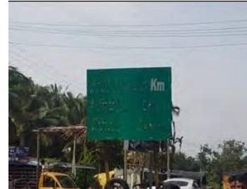
Fig. 15: Poor condition of sign Board at ch.190.100 Km
