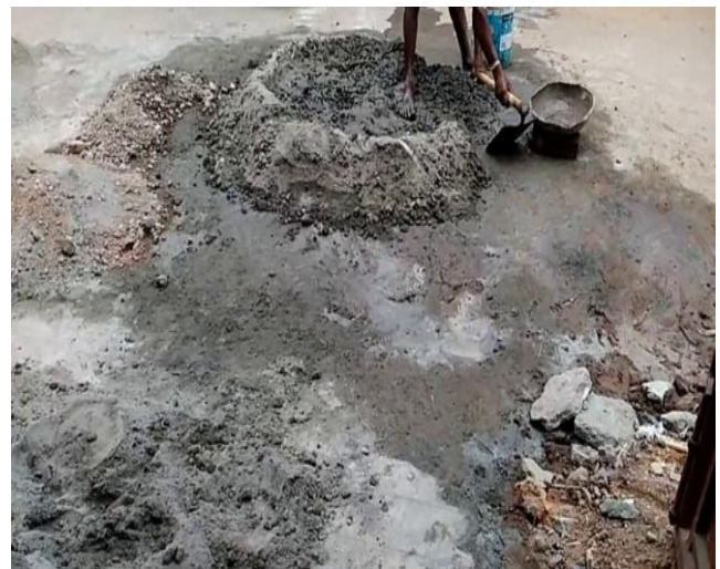
Fig 2: Mixing of concrete
