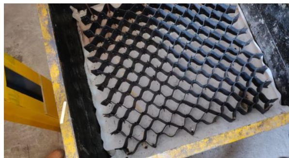
Fig. 5. Expanded Rubber cell installed on the Geotextile over subgrade
