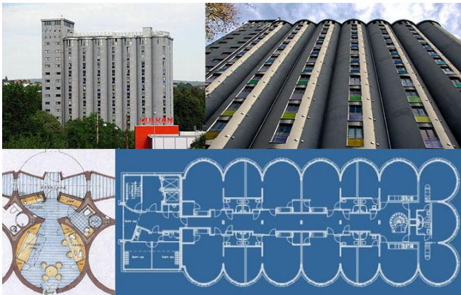
Fig. 2 Student Housing Complex, HRTB Arkitekter AS
