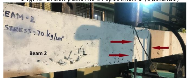
Fig.4c Crack patterns in specimen 2
