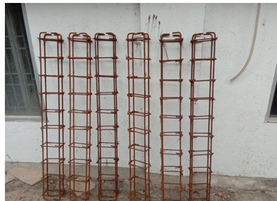
Fig 2 Reinforcement for Beam
